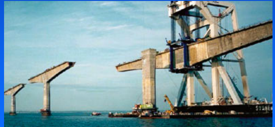
| Confederation Bridge – Canada
