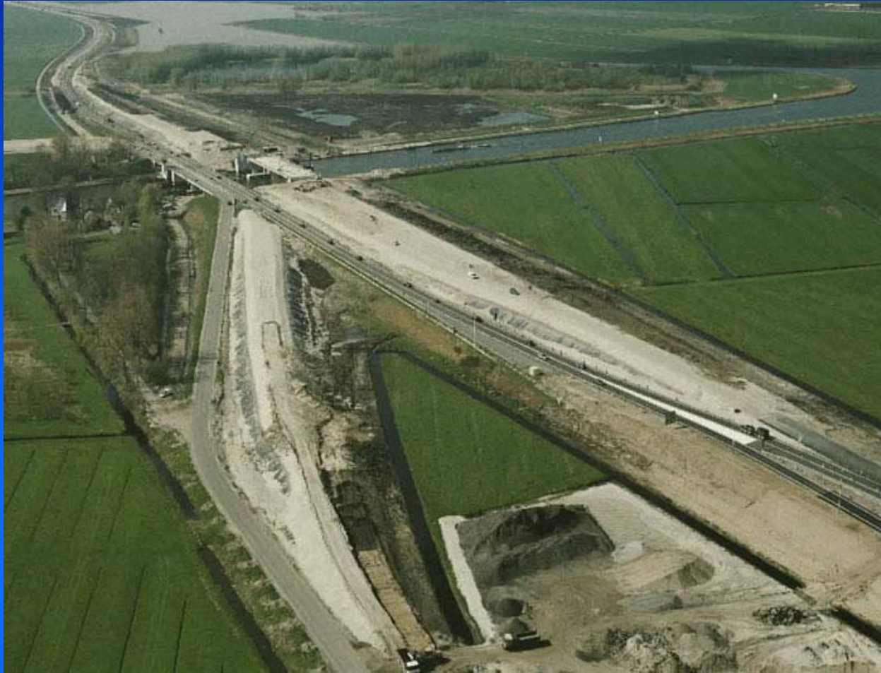
Wâldwei: aquaduct, widening of existing road and maintenance
