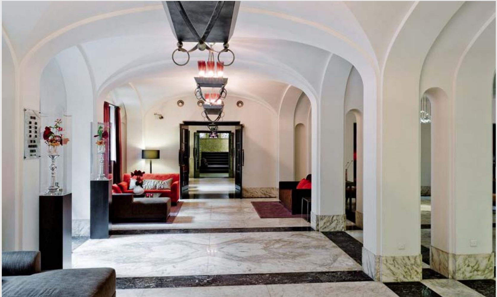
Renovatie interieur hotel The Grand, Amsterdam
